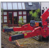
Level operation on uneven sites
